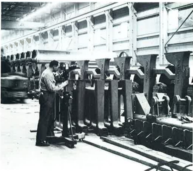
Inspecting critical alignment of rollers on a paper machine with a K&E Jig Transit. In many cases, present-day tolerances would be impossible without optical devices.
