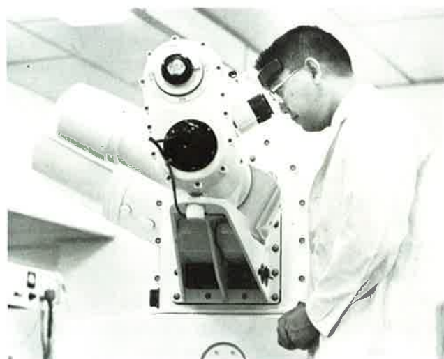
A major research and development project of the 1960's was the K&E missile-tracking cinetheodolite.
